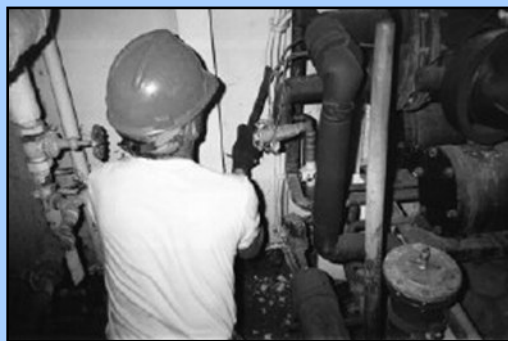
Frank Wright attacks the rusting paint during restoration of the Glacier.
